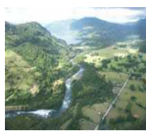
Choshuenco 128 MW Chile
