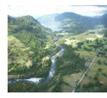
Choshuenco 128 MW Chile
