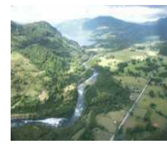
Choshuenco 128 MW Chile
