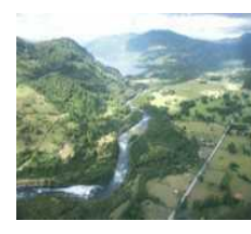
Choshuenco 128 MW Chile
