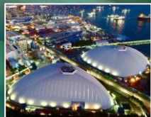
Bocamina II September 2022
