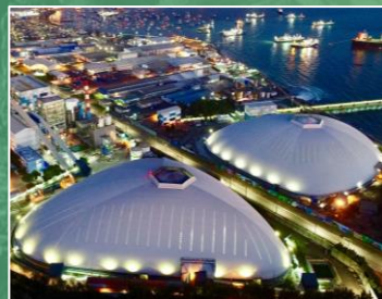
Bocamina II September 2022
