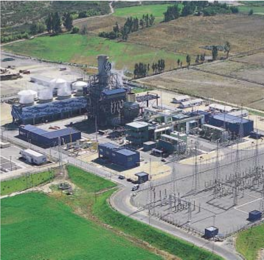
SAN ISIDRO COMBINED-CYCLE THERMAL PLANT, CHILE
