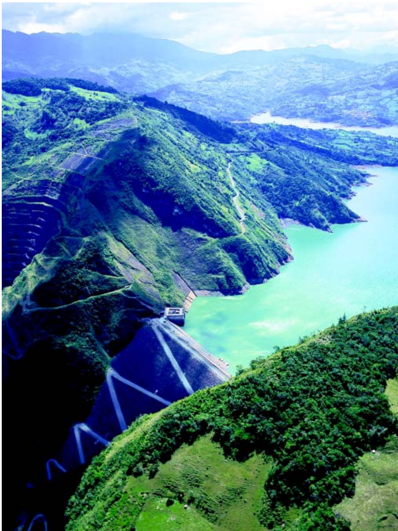
UBALÁ RESERVOIR, EL GUAVÍO HYDROELECTRIC POWER PLANT, COLOMBIA
