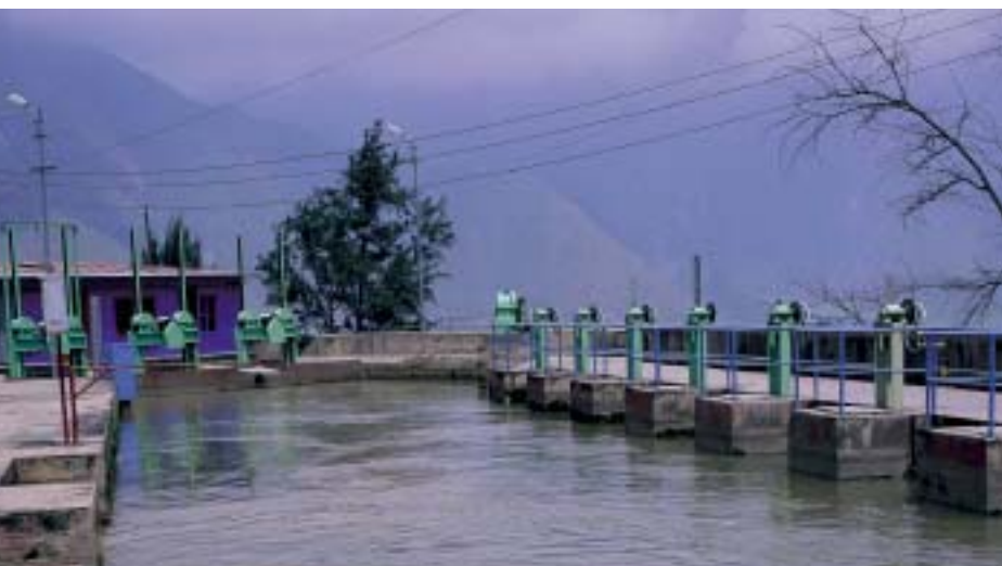
CHAMBER OF CALLAHUANCA POWER PLANT, PERU
