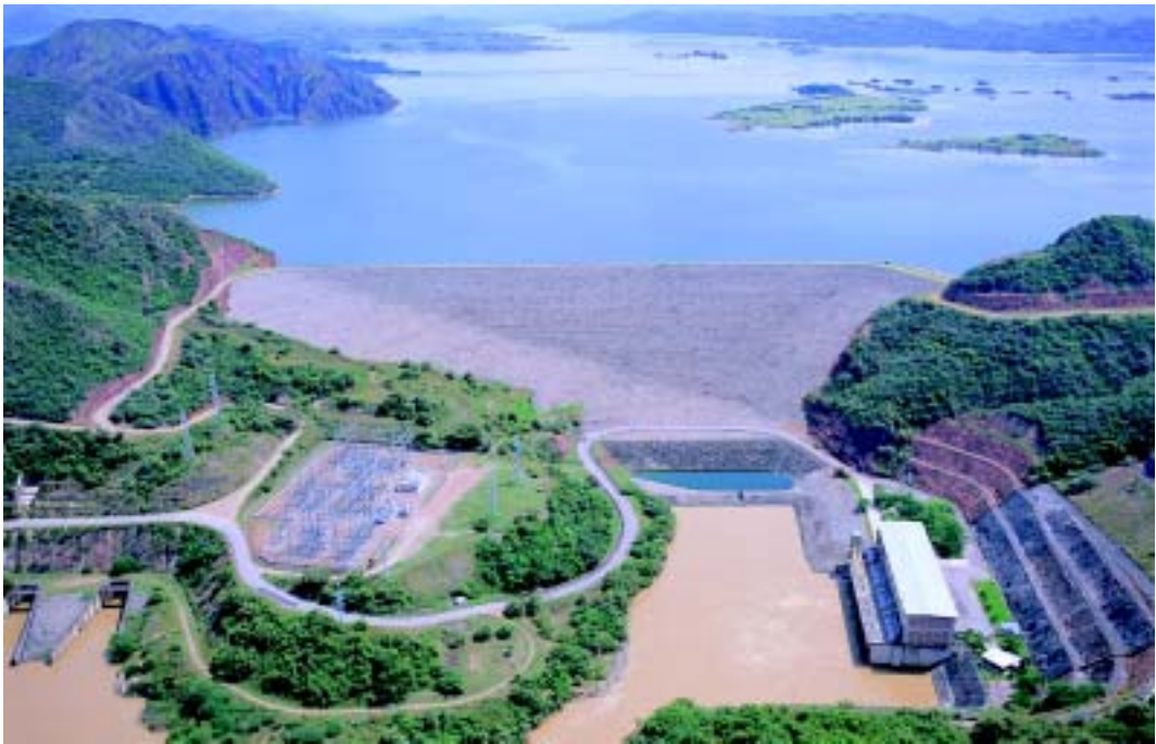
BETANIA HYDROELECTRIC PLANT, COLOMBIA
