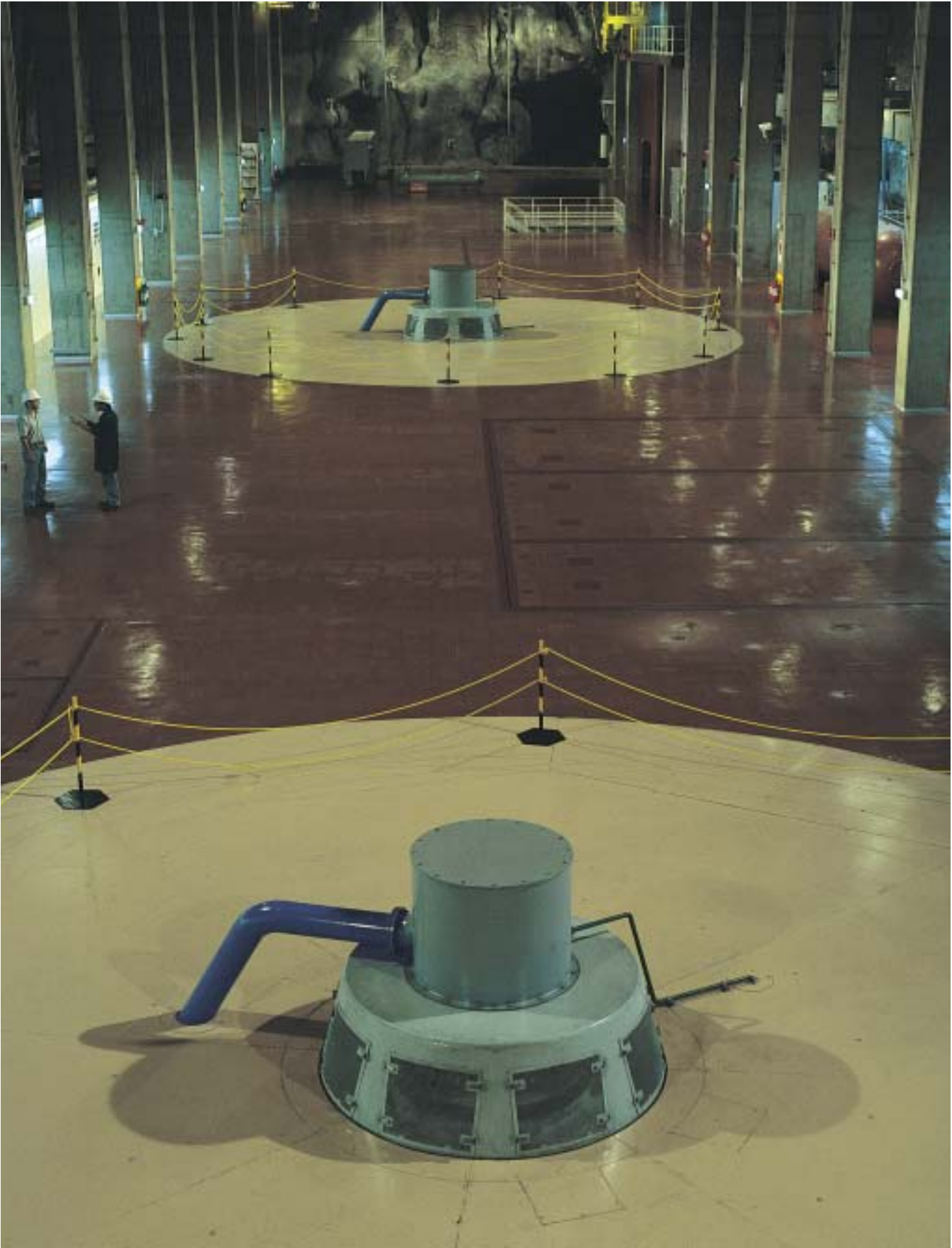
UNDER GROUND POWER HOUSE OF PEHUENCHE HYDROELECTRIC POWER PLANT, CHILE
