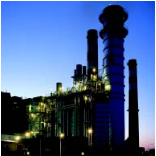
CBA COMBINED-CYCLE THERMAL PLANT, ARGENTINA
