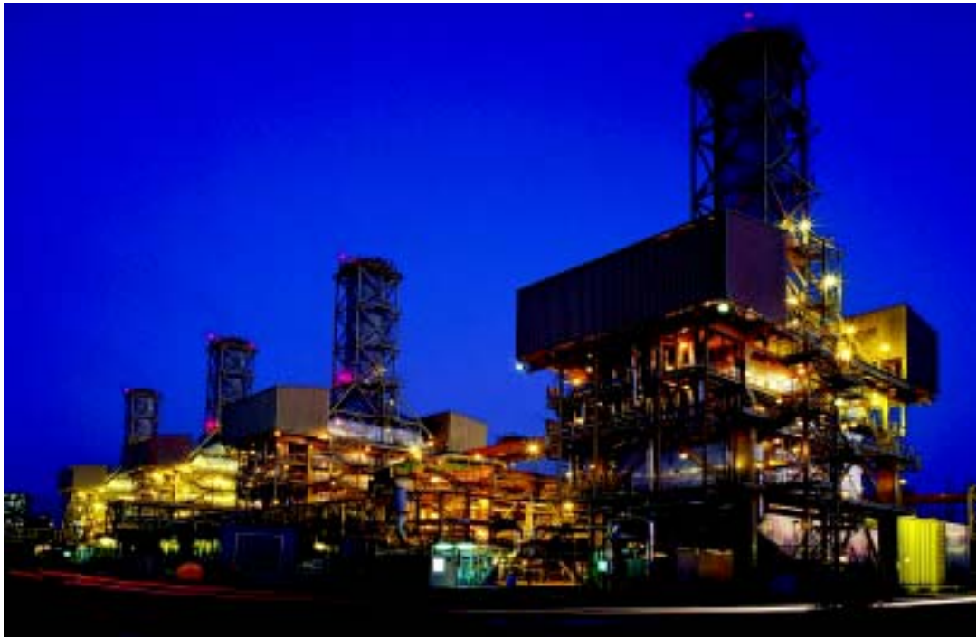
ATACAMA COMBINED-CYCLE THERMAL PLANT, CHILE
